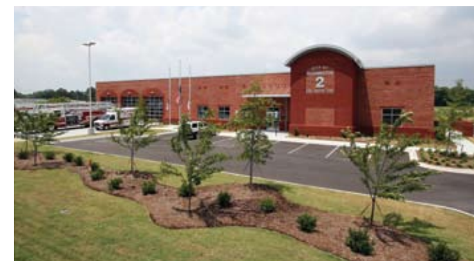
washington fire/rescue/ems station
