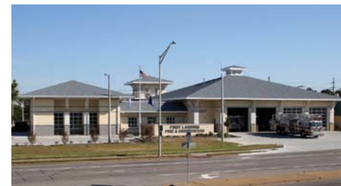
virginia beach fire/rescue station ACA Architects + SCN Architects
