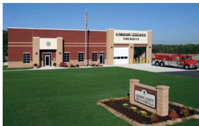
gordon county fire substation
