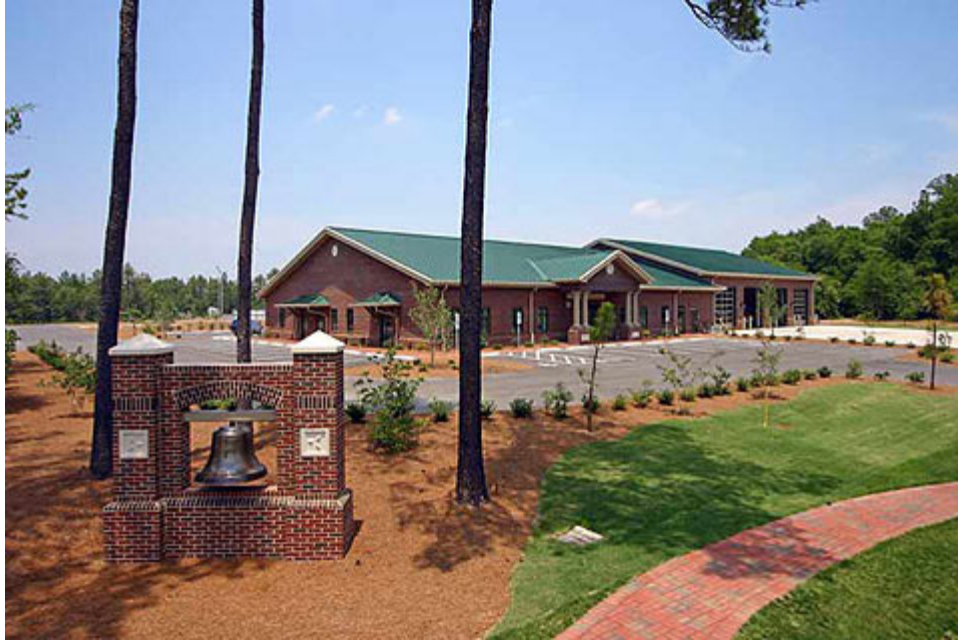
The Pinehurst Fire Station was planned with adequate space on all sides for future additions.
